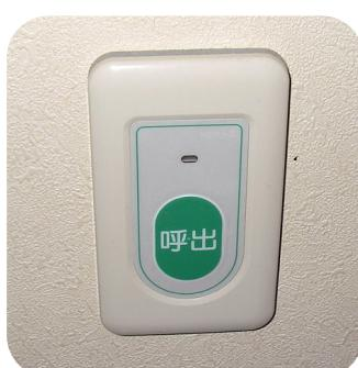
The button with 呼び出し (call) is an emergency button. If you feel ill or are injured, press the button for assistance. Sometimes, people press this button by mistake to flush the toilet. Try to remember that 呼び出し (call) is an emergency button.
